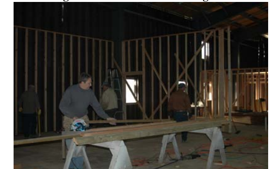
Rod Reiger & Ron Tennison building a wall
